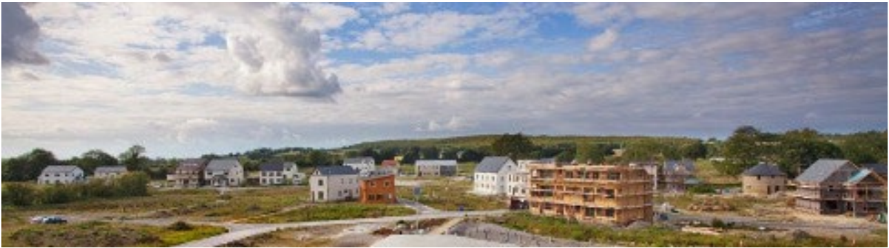
Figure 4 - New efficient buildings at “Eco-Village”, North Tipperary
