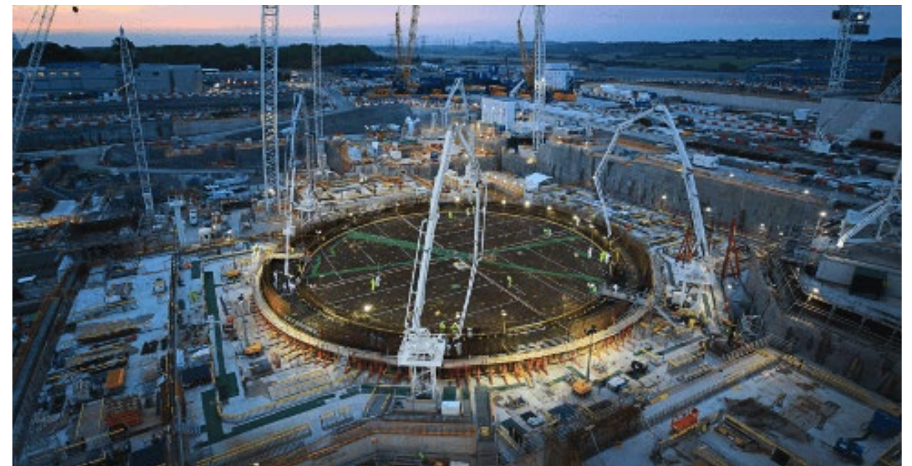
Figure 5 - Construction of Hinkley Point C Power Station, Somerset. [Credit: EDF Energy]
